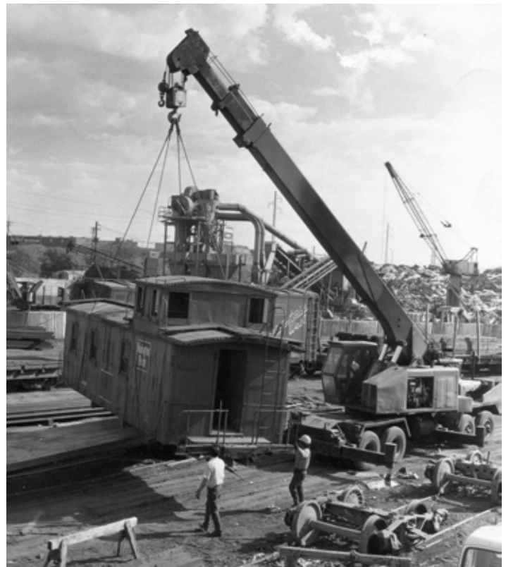
Right: In May 1974, the caboose is being loaded on a flatbed trailer to be transported to Al Jackson's property in Loveland. The crane operator isn't using spreader bars, and there was some minor damage to the siding and eyebrow boards as a result. Below: The caboose is on a train at South Denver in 1958. Both photos, Al Jackson collection.
