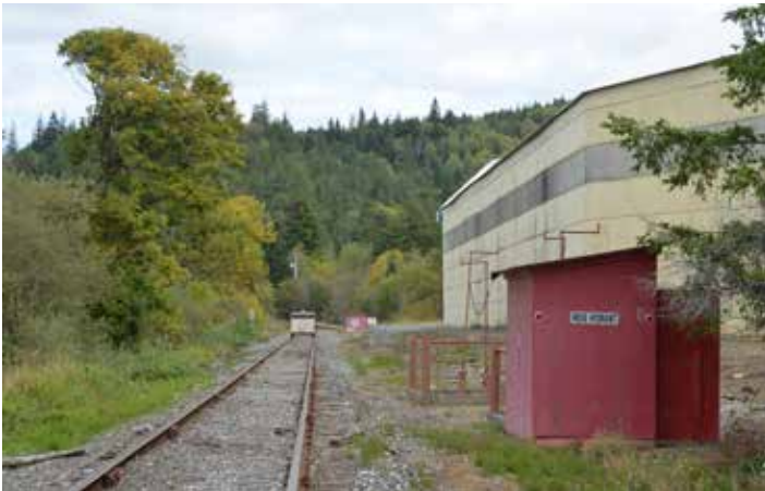
Every 200-300 feet in lumber loading areas, there is a red painted fire hose & hydrant shack along the rails. Each one is just slightly larger than an outhouse.
