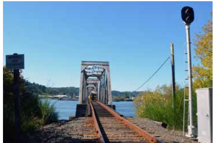
The northern approach to Reedsport Drawbridge at milepost 739.5.
