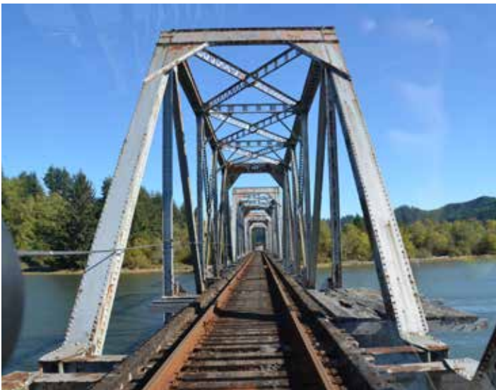
MP 739.6, the Reedsport Drawbridge crossing the Umpqua River.
