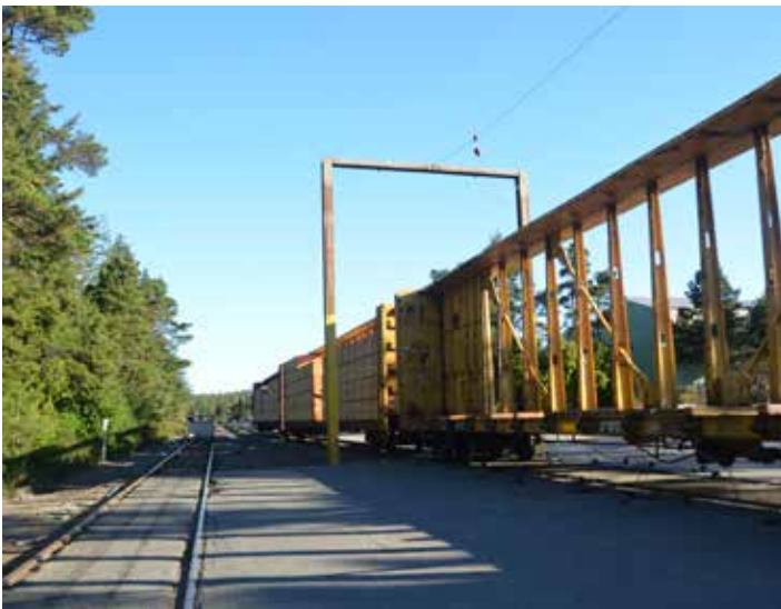
Lumber loading siding (2980') at Hauser, milepost 759.4. The rectangular frame is not a tell-tale for tunnel clearance; the cable running between two frames is a tie-in point for a worker in a body harness with lanyard. This is an approved method of fall prevention when walking across the tops of cars, something still allowed while loading and unloading.
