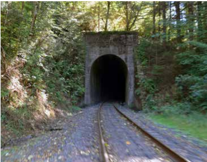
Southern portal to tunnel 15 (2143') at milepost 721.5.
