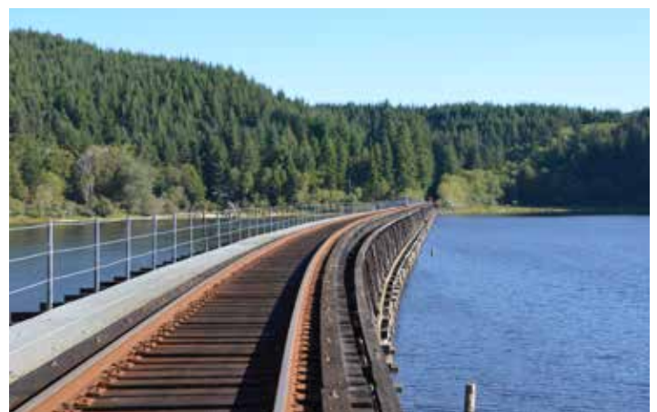
Milepost 750.7, another long trestle crossing North Tenmile Lake.
