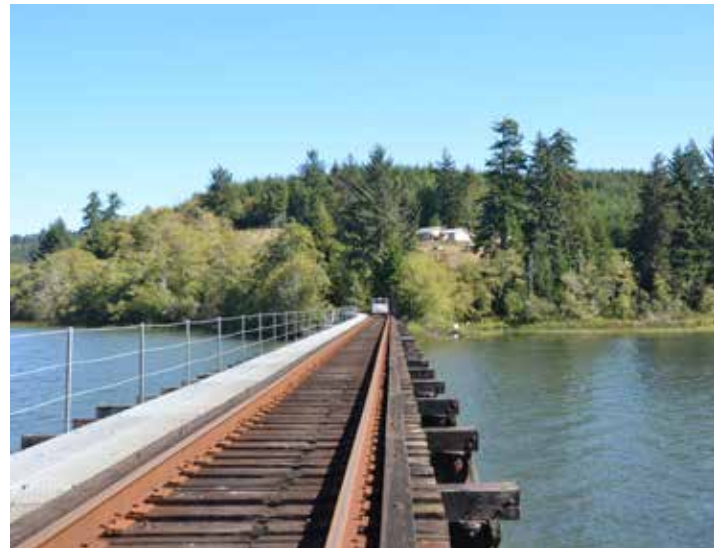
Milepost 726.5, Bridge near the station of Canary.
